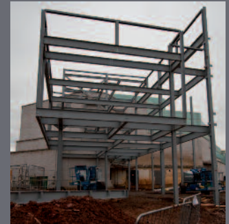
Dec 08 - steelwork built for extension
