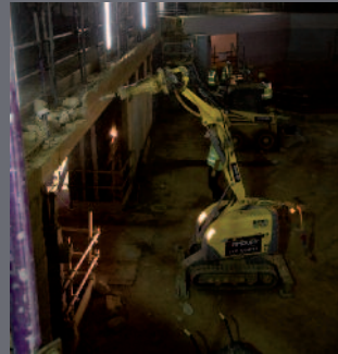
Sept 08 - demolition of interior
